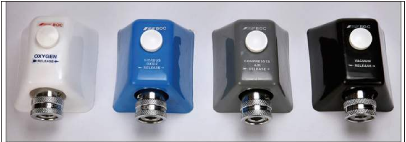
Figure 3 – Terminal wall outlets from medical gas pipelines at point of use
