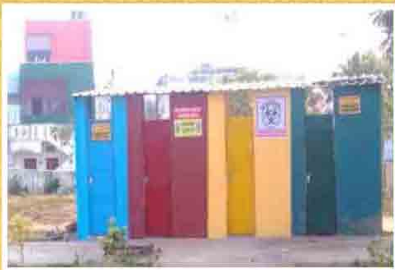
AH Atmakur, Andhra Pradesh
